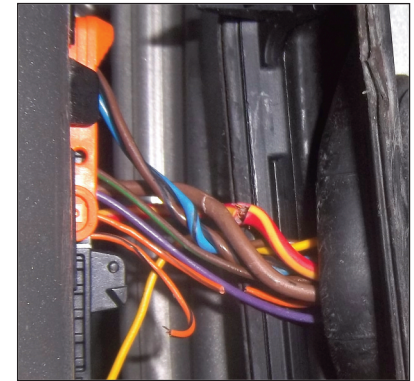
The wiring had broken under cover of the rubber boot causing the window failure
