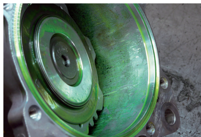
Figure 2: Too much contrast agent in the compressor oil
