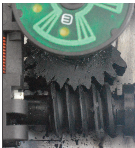
CIPOS gear, worm gear and motor failure. A complete gearbox is required with failures of this nature.
