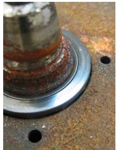
Destroyed mechanical face seal – the sliding surface was corroded by foreign particles
