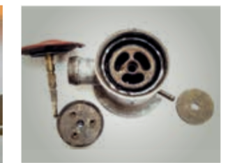
Pneumatic secondary air valve: Damage (to diaphragm and valve head) due to condensate
