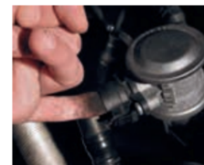
Simple inspection of secondary air valve
