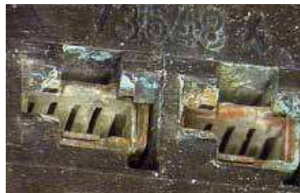
Coupling with traces of moisture and corrosion
