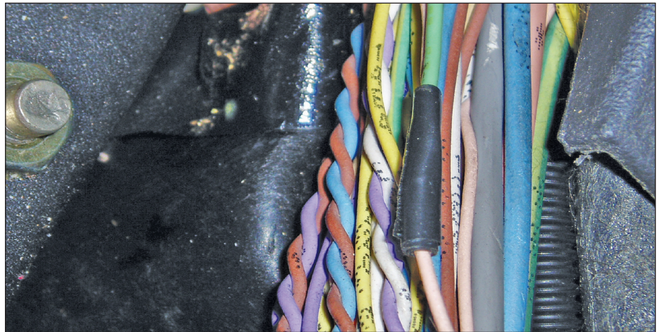
The cause of the intermittent fault: a partially cut wire that would only act up when the driver put their foot on a plate that covered the wiring loom
